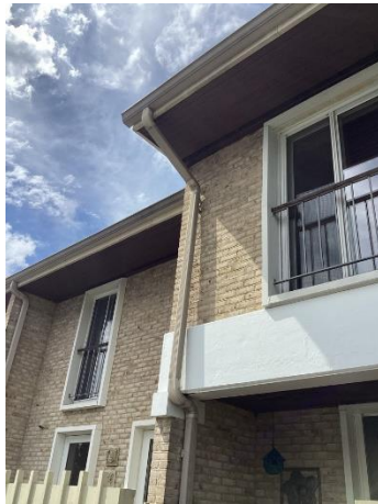
Gutters and downspouts
