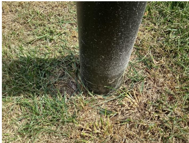
Finish deterioration
