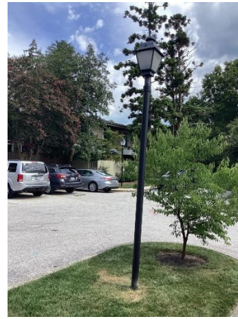
Leaning light poles and fixtures
