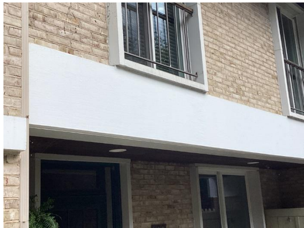
Soffit and fascia overview
