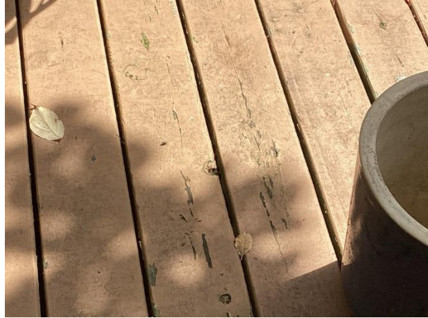
Finish deterioration
