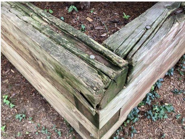
Wood deterioration
