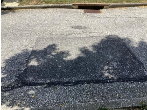
Patches and repairs
