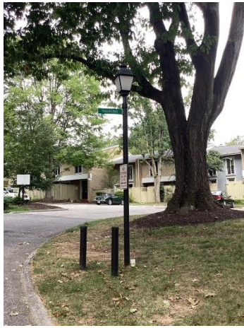
Light poles and fixtures
