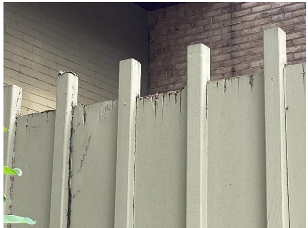
Wood deterioration
