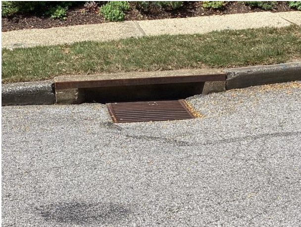
Catch basin overview
