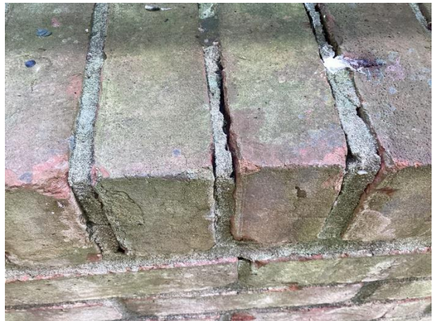
Mortar deterioration
