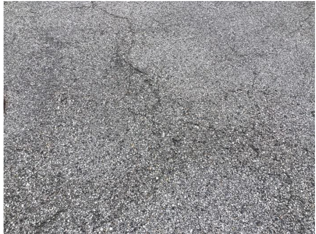
Pavement deterioration
