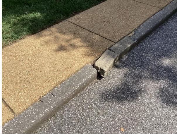
Concrete spalls
