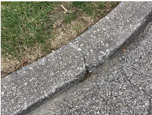
Concrete cracks
