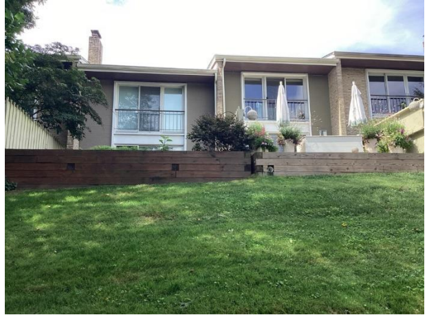
Timber retaining walls overview
