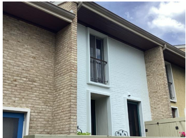
Masonry walls overview
