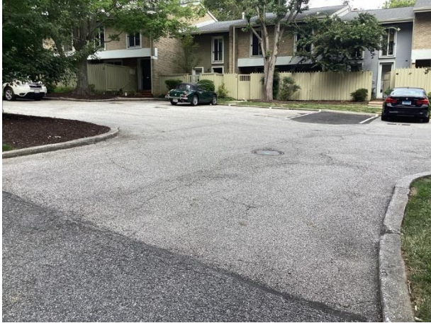
Asphalt pavement overview
