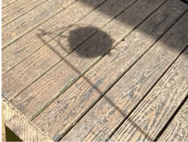
Finish deterioration
