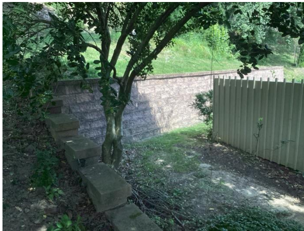
Masonry wall north of Palmer Green Court
