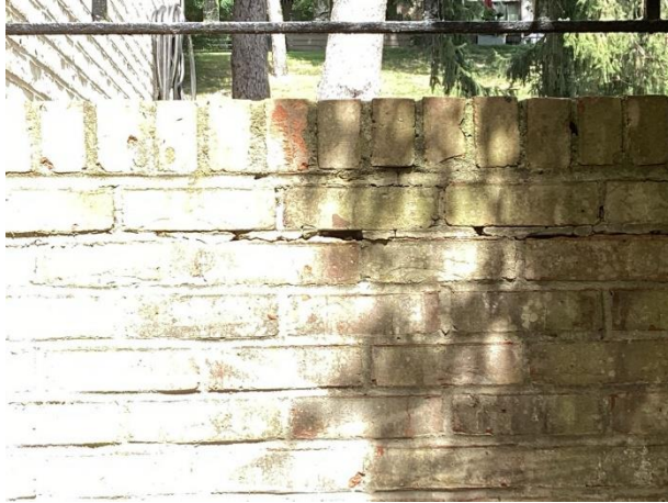
Mortar deterioration
