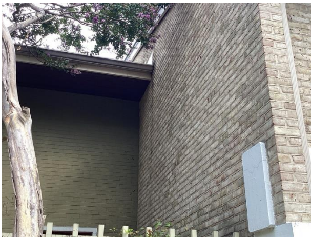
Masonry walls overview
