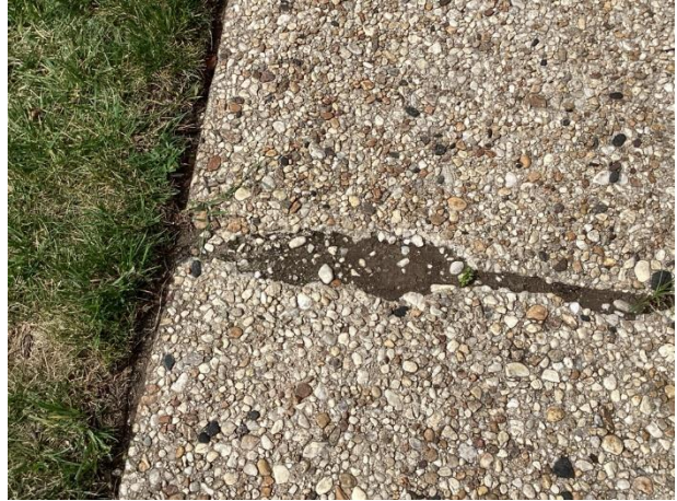
Concrete spalls
