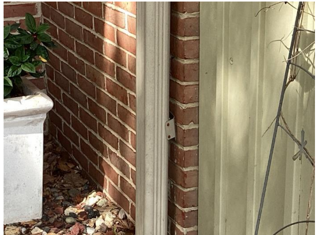
Rusted fasteners
