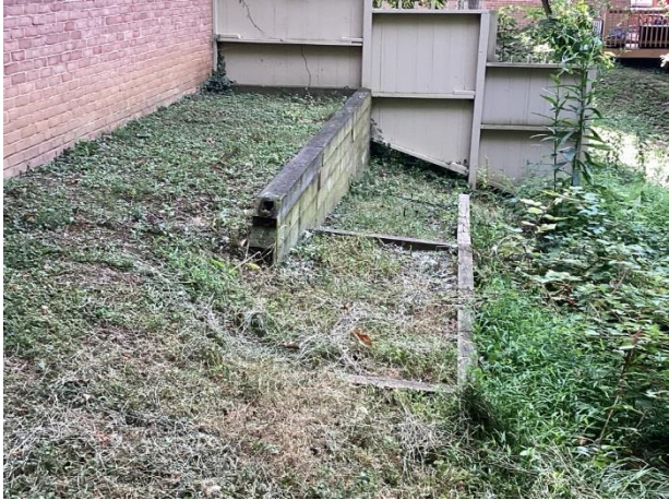
Timber retaining walls overview
