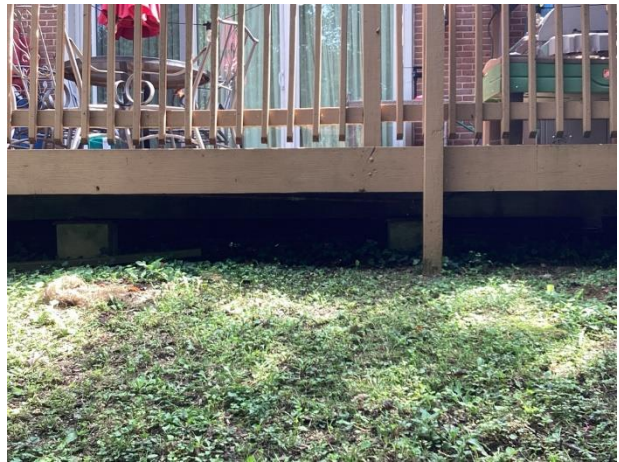
Deck underside overview
